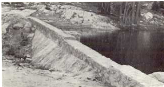
Stream flow maintenance dam at the outlet of McClure Lake
